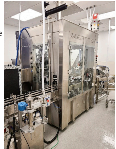
Tri-Pac Line 7 – Foam & Spray Aerosol Filling
